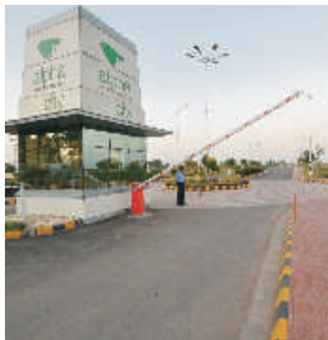
Secured entrance to AIC Fatehabad
