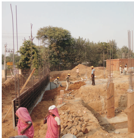
Structural work of shopping arcade in progress
