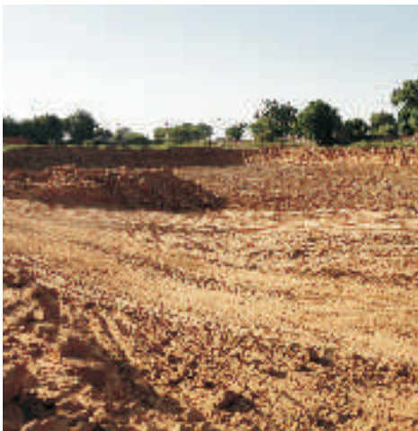
Excavation work being carried out at GO 84
